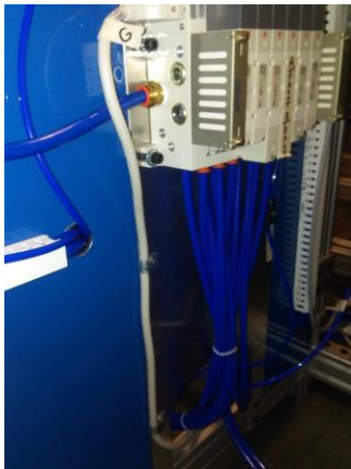
Shows G cable to power block, and airlines.
